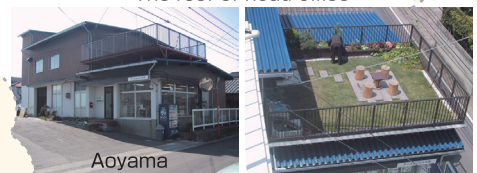
The roof of head office
